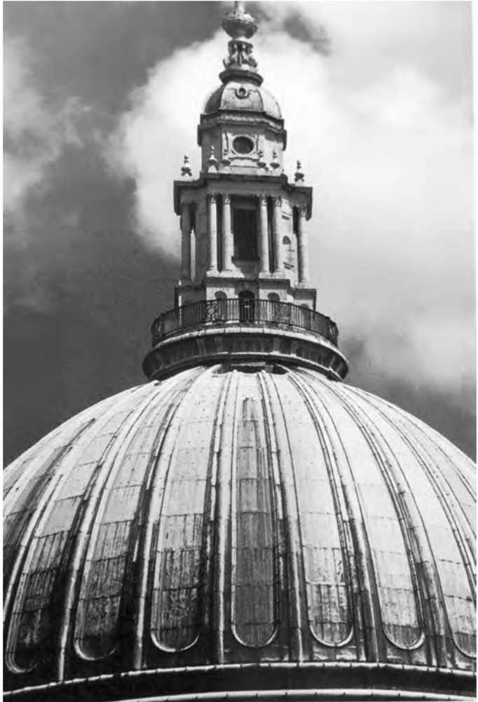
DOME OF ST. PAUL'S CATHEDRAL
